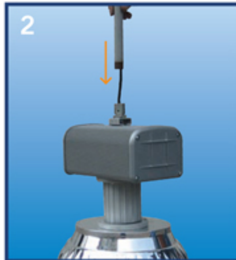
Attach conduit to Meyers Hub
