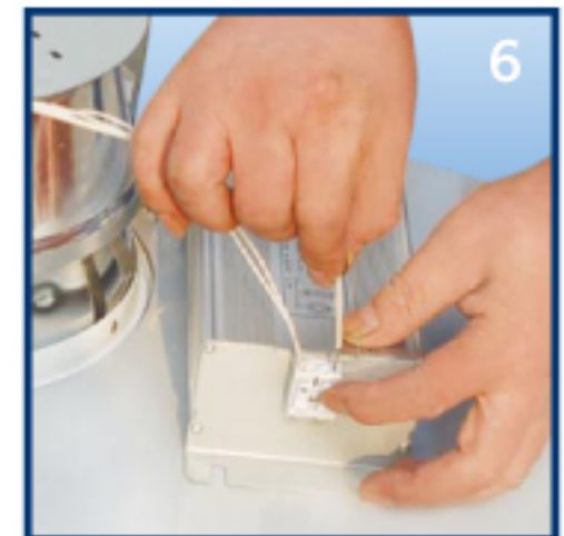
Connect the lamp wires to the ballast
