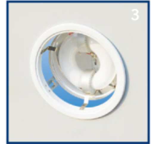
Picture of inserted fixture
