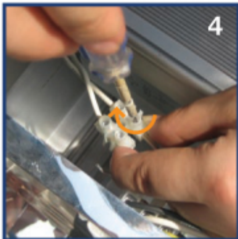
Tighten wires
